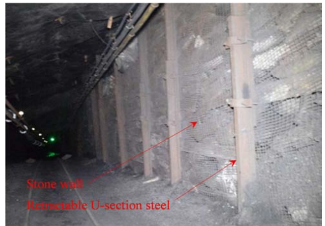
Figure 15. Effect of secondary gob-side entry retaining.
